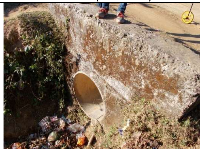
HP Culvert (Ch. 148.698 km)
