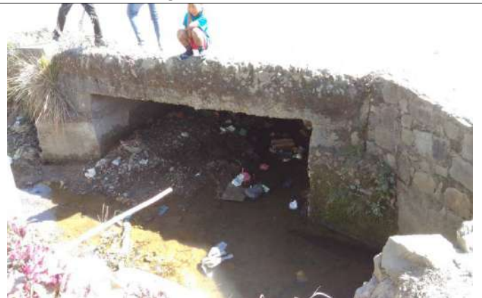
Slab Culvert (Ch. 4.061 Km)
