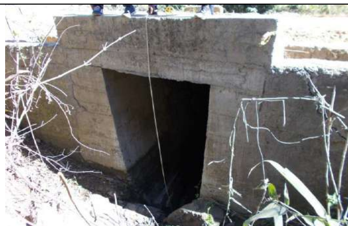
Slab Culvert (Ch. 44.482 Km)
